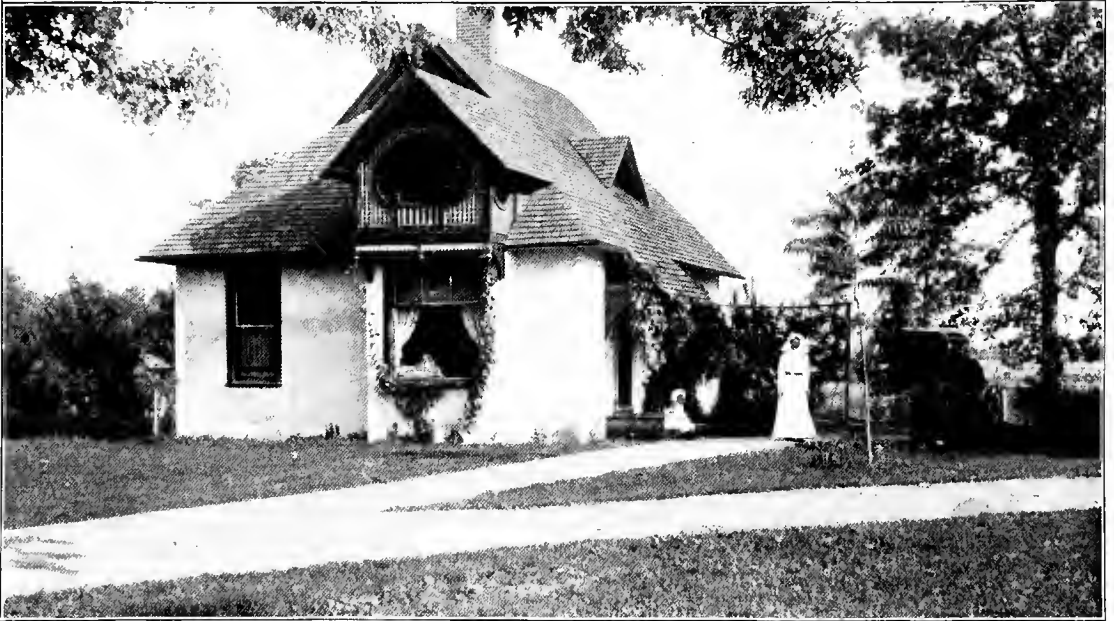
FIG. 218—A PLASTERED HOUSE.
